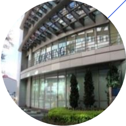
Corning Research Center Taiwan Hsinchu, Taiwan
