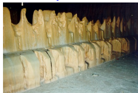
refractory corrosion
