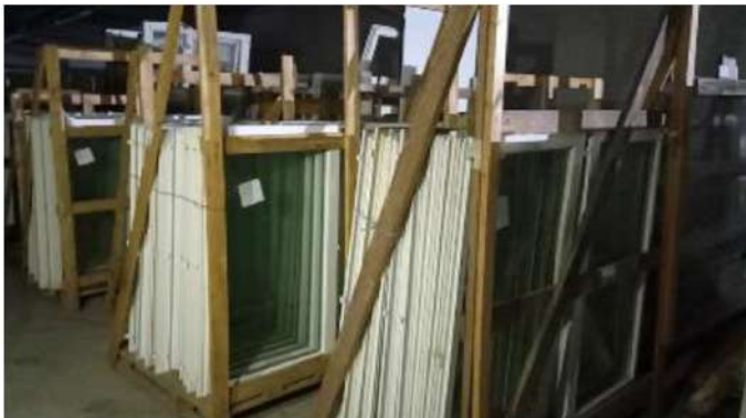
Careful removal and storage to preserve the integrity of the glazing
