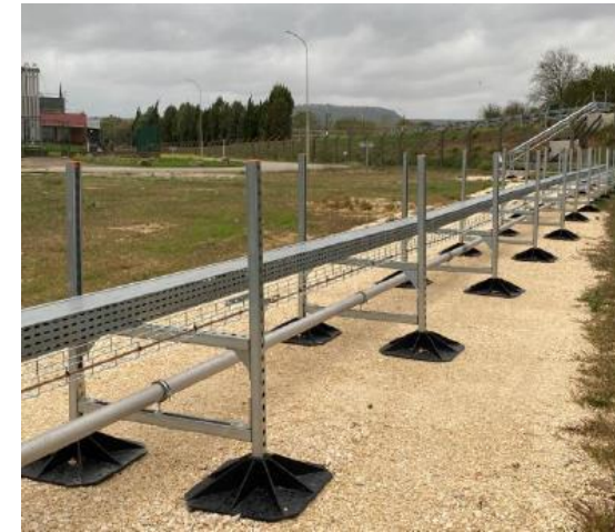
H 2 piping (500m) – outside/inside plant
