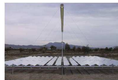
Tour de Fresnel \eta \approx 9-11\%
